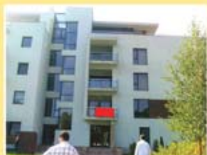
Apartament 3 cam. complex Băneasa, imobil 2008
